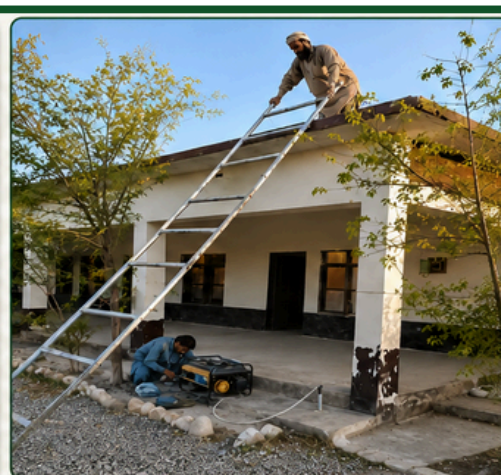
Zhob-Repair and rehab of FCPS Murgha Kibzai
