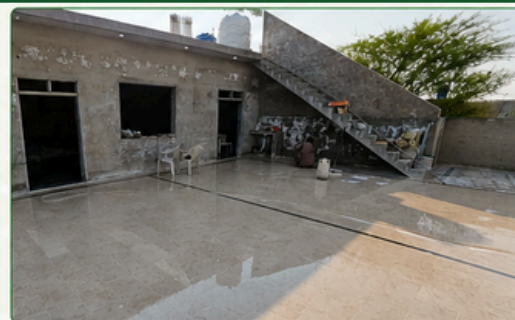
Sibi -CONSTRUCTION OF PRESS CLUB
