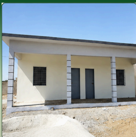
Panjgur- CONSTRUCTION OF 2 CLASSROOMS
