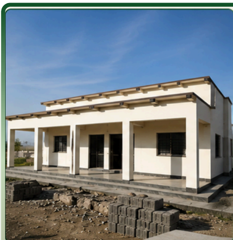
Panjgur -Repair and Renovation of GBPS Mola Dad Village
