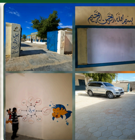
Panjgur-REPAIR AND RENOVATION GBMS KHUDABADAN, BUG WARD
