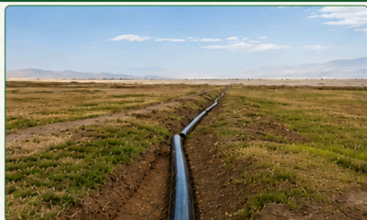
Sherani -PVC Pipe Line (2000 Rft)
