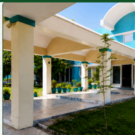
Sibi-Provision and fixing of solar system at circuit house
