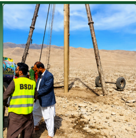
Pishin -Construction of wss for killi gawal, tehsil karezat
